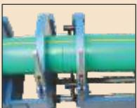
**Machining:** If the gap between the two ends of pipe exceeds 0.5 mm at any point then machining is recommended.
